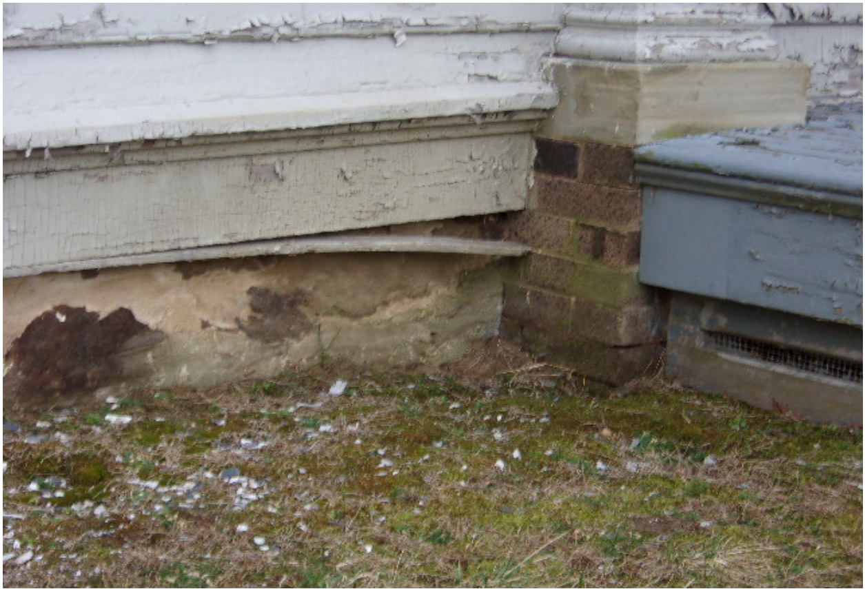
Photo 18- West Elevation Wood Damage Detail
