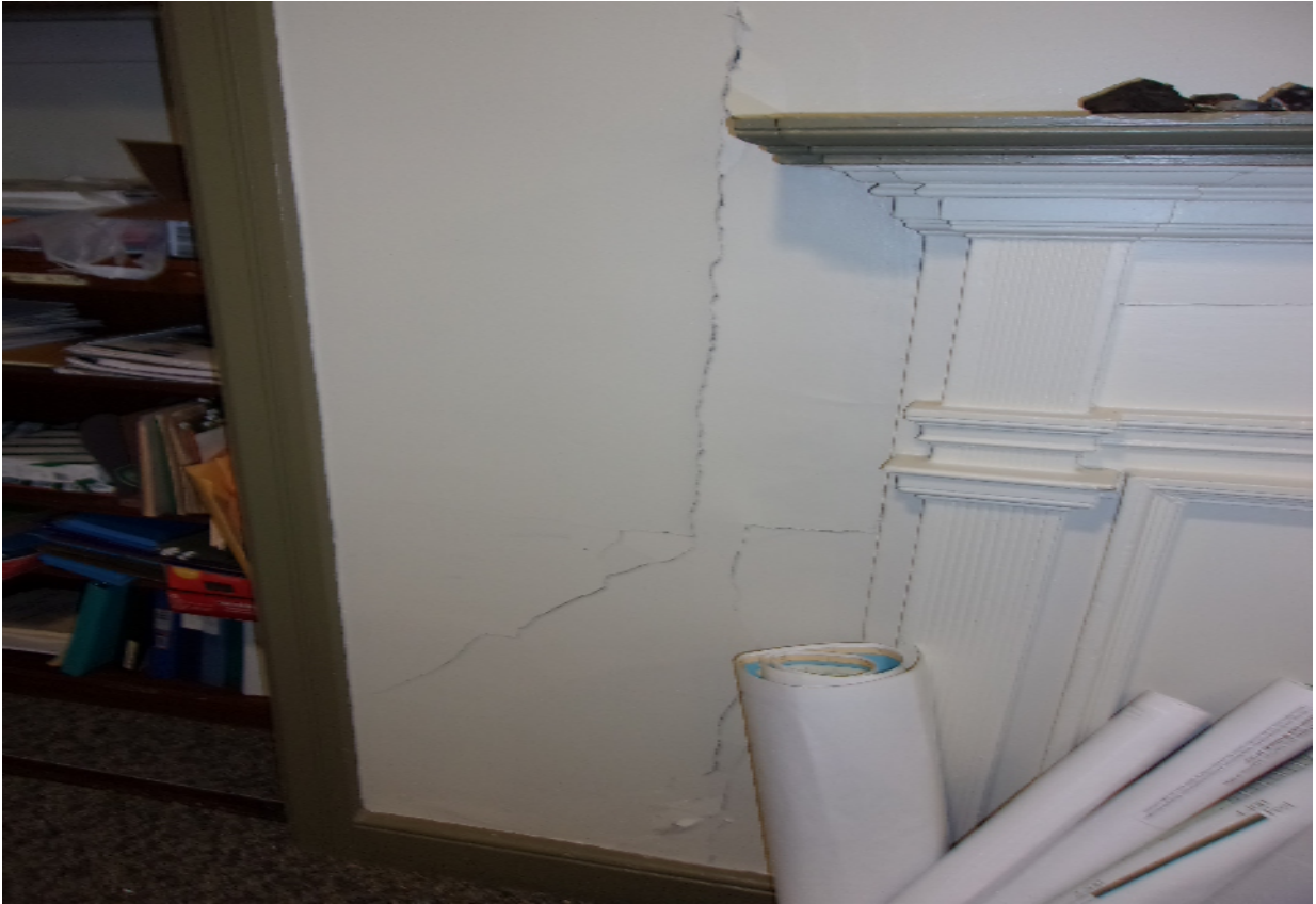
Photo 11-Interior Structural Cracks
