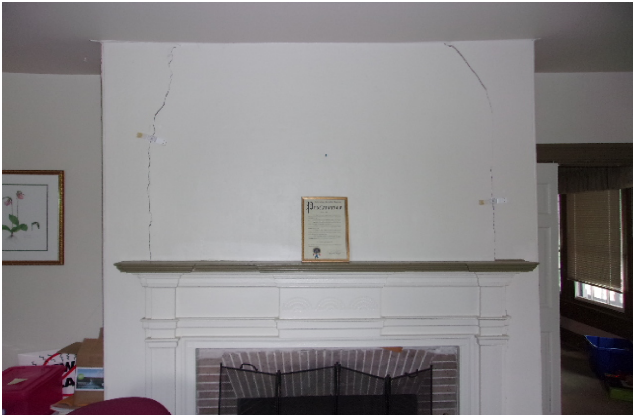
Photo 15-Interior Structural Cracks
