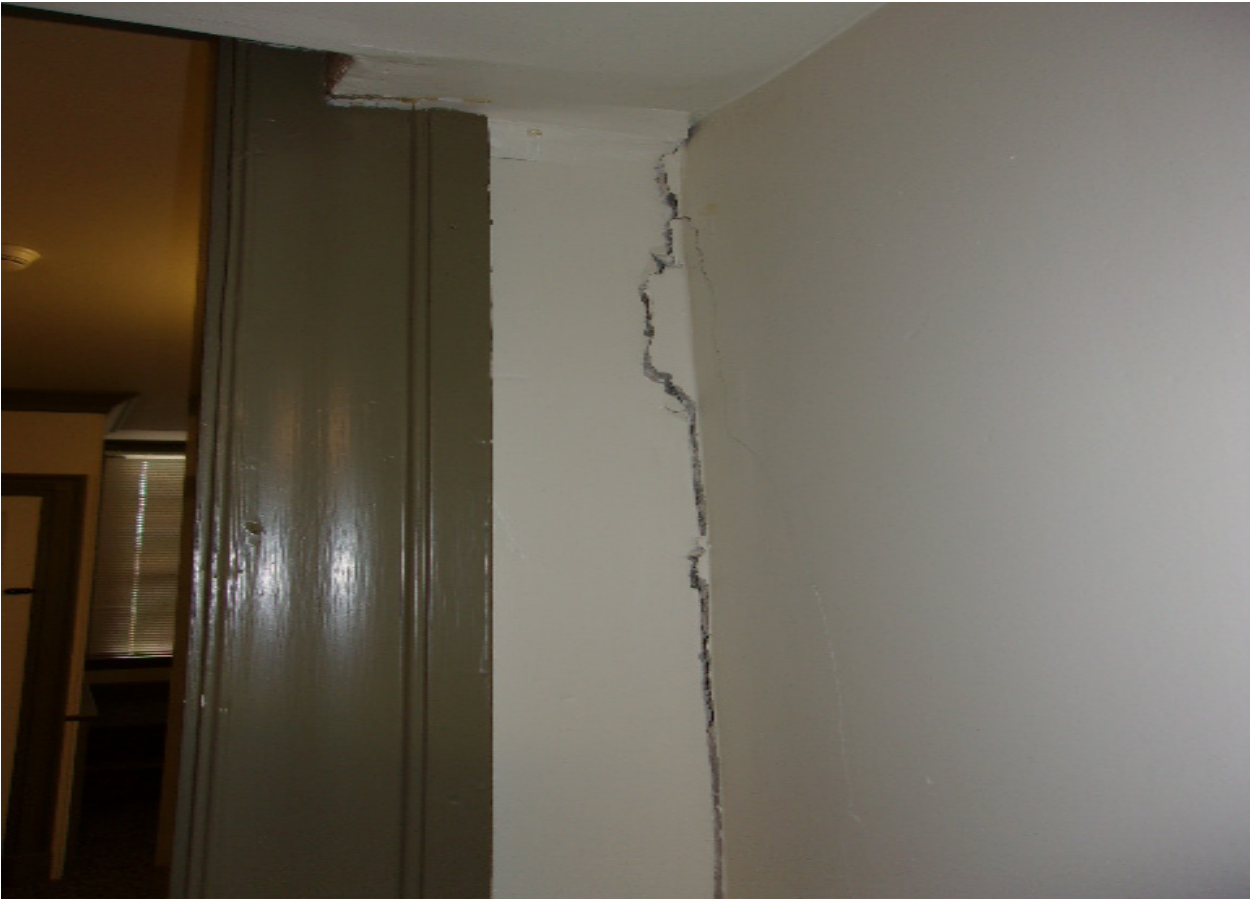
Photo 12- Interior Structural Cracks
