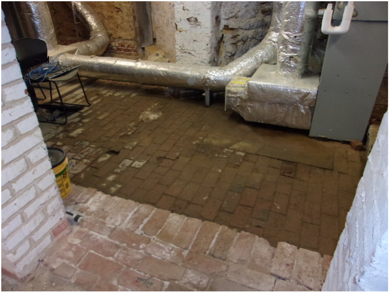
Photo 22- Water Saturated Brick Cellar Floor
