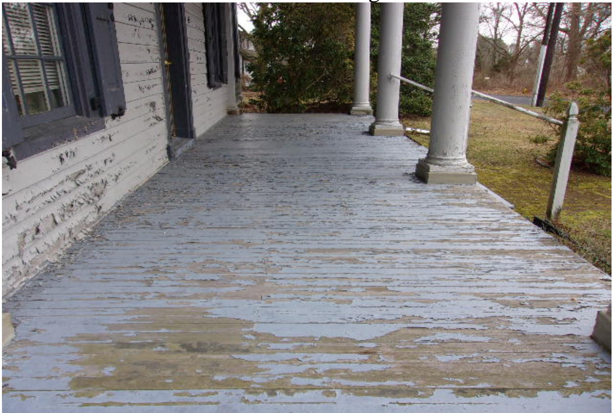
Photo 19-West Entrance Porch Damage Overview
