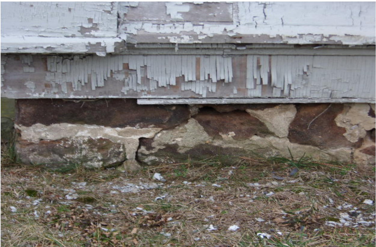
Photo 17-Fenwick Ironstone Foundation Crack and Wood Damage
