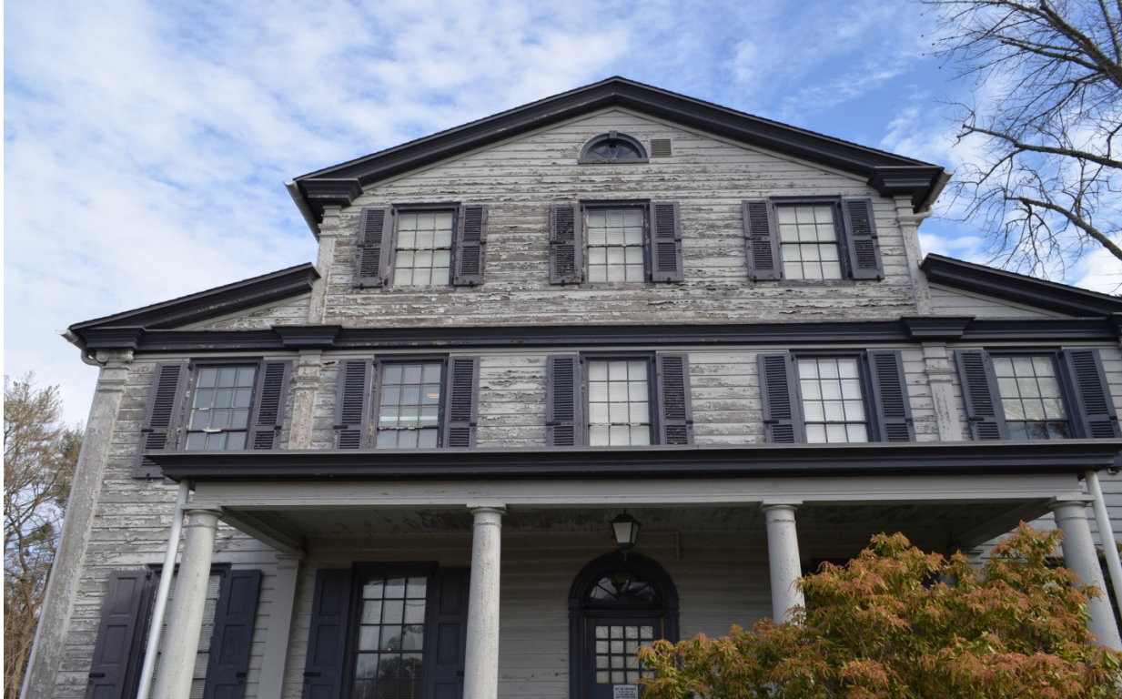
Photo 5-West Elevation/ Damage Overview
