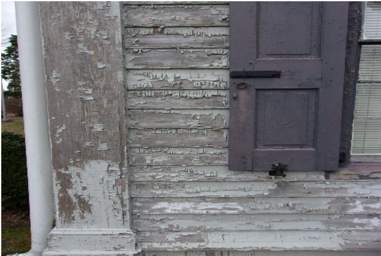
Photo 20-West Elevation Damage Detail
