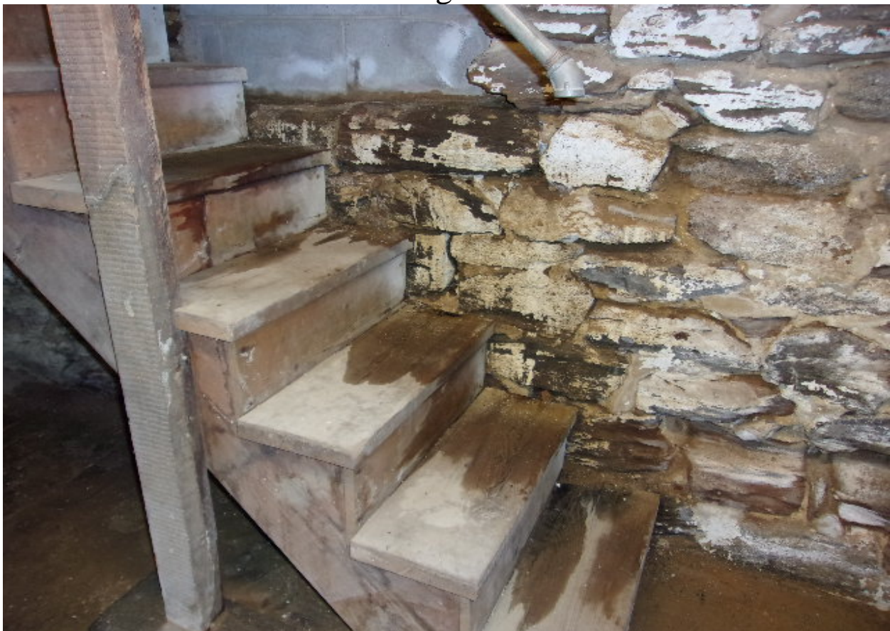
Photo 21-Water Seepage from North Cellar Wall
